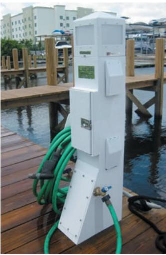
Power pedestal enclosures for marinas are manufactured using a variety of materials from lightweight composites to marine grade aluminum and stainless steel. The type of materials
